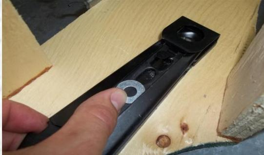
3-Align the screw into the washer.
